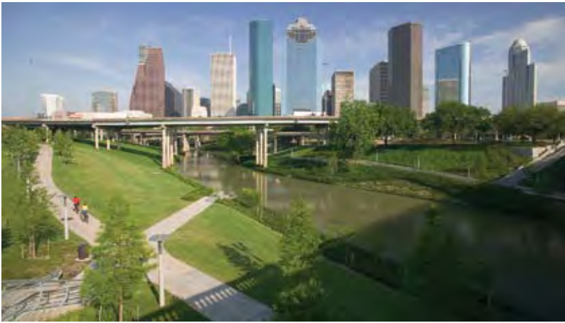
Brays Bayou (top) and Buffalo Bayou Promenade (above) in Houston are prime examples of how complementary green and gray infrastructures can restore river morphology to create active space while also providing flood protection.
