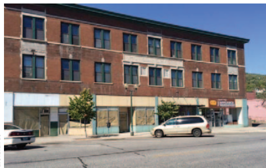
The Esmond Building on West Superior Street incorporates residential and commercial uses.
