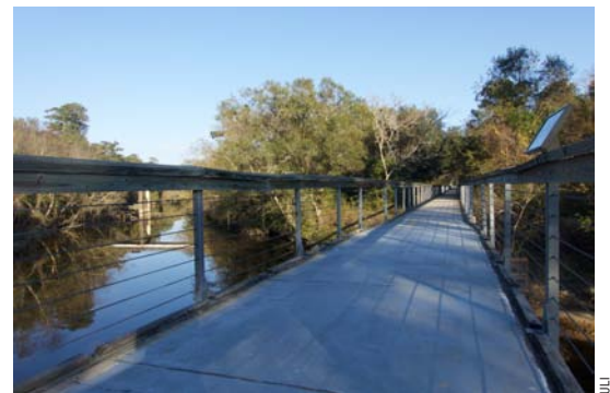
View of Tammany Trace multimodal trail over the Bogue Falaya in Covington.
