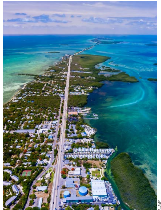
The "spine" created by deposited limestone in the Florida Keys is higher than surrounding terrain and therefore makes an attractive area for infrastructure.
