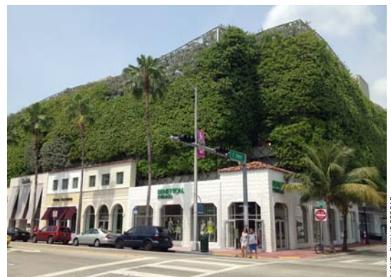
Ballet Valet, a parking garage in Miami Beach, uses green walls to capture rainwater before it hits the ground.
