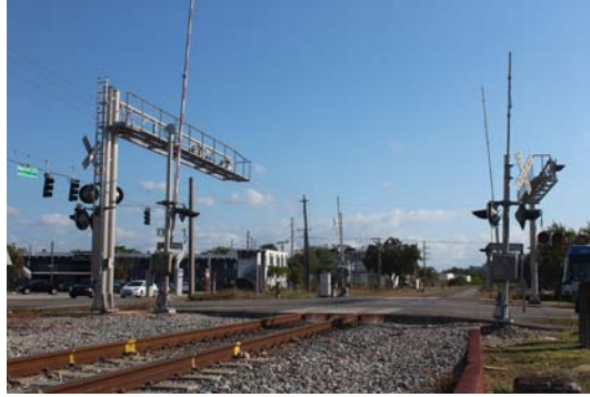
The site for the proposed Tri-Rail Coastal Link station is surrounded by a low density of uses, providing an opportunity for housing and economic development.
