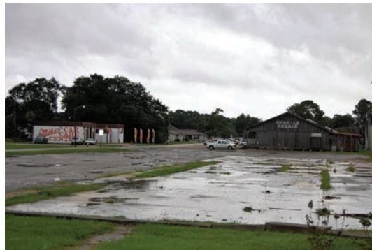
During the week of the panel, nuanced flooding was observed even during an average rain event.
