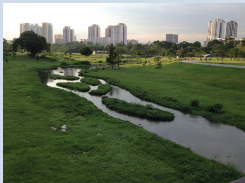
The Kallang River was removed from its concrete encasing and now can widen up to 330 feet in flood conditions, increasing conveyance by 40 percent.
