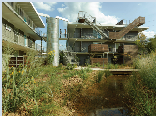
A bioswale helps filter the runoff at ECO Modern Flats in Fayetteville, Arkansas.
