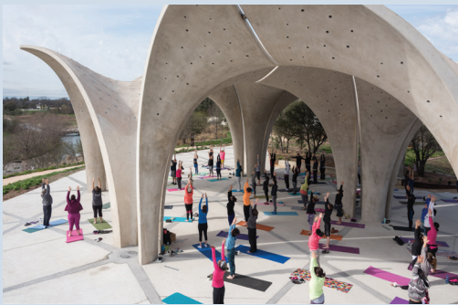
Weekly yoga sessions are a part of the events and programming schedule that keep the park engaged with its community. Here a yoga class gathers under the central pavilion, which serves as a water management feature.
