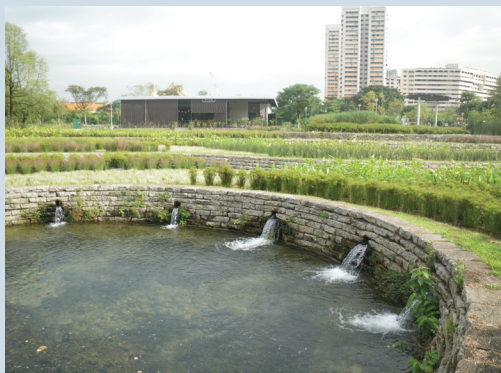
The cleansing biotope helps filter the water before it is returned to the drainage system in the park.
