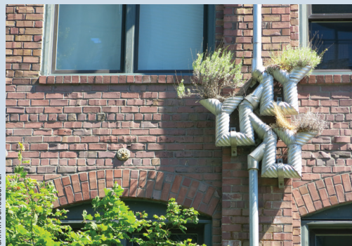
Environmental sculptor Buster Simpson designed several pieces for Vine Street, including this feature on a building facade, which helps filter rain and stormwater runoff.
