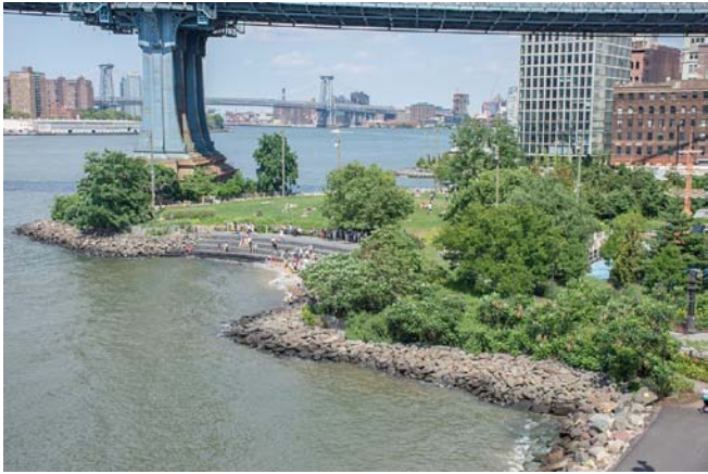
An example of terraced steps with riprap in Brooklyn Bridge Park.
