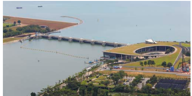
The London Thames Barrier (top) and the Singapore Marina Bay Barrage (above) are large-scale examples of tidal gateways. A smaller-scale tidal barrier at the mouth of the Miami River could eliminate the significant impacts of surge flood for the residential communities along the river.
