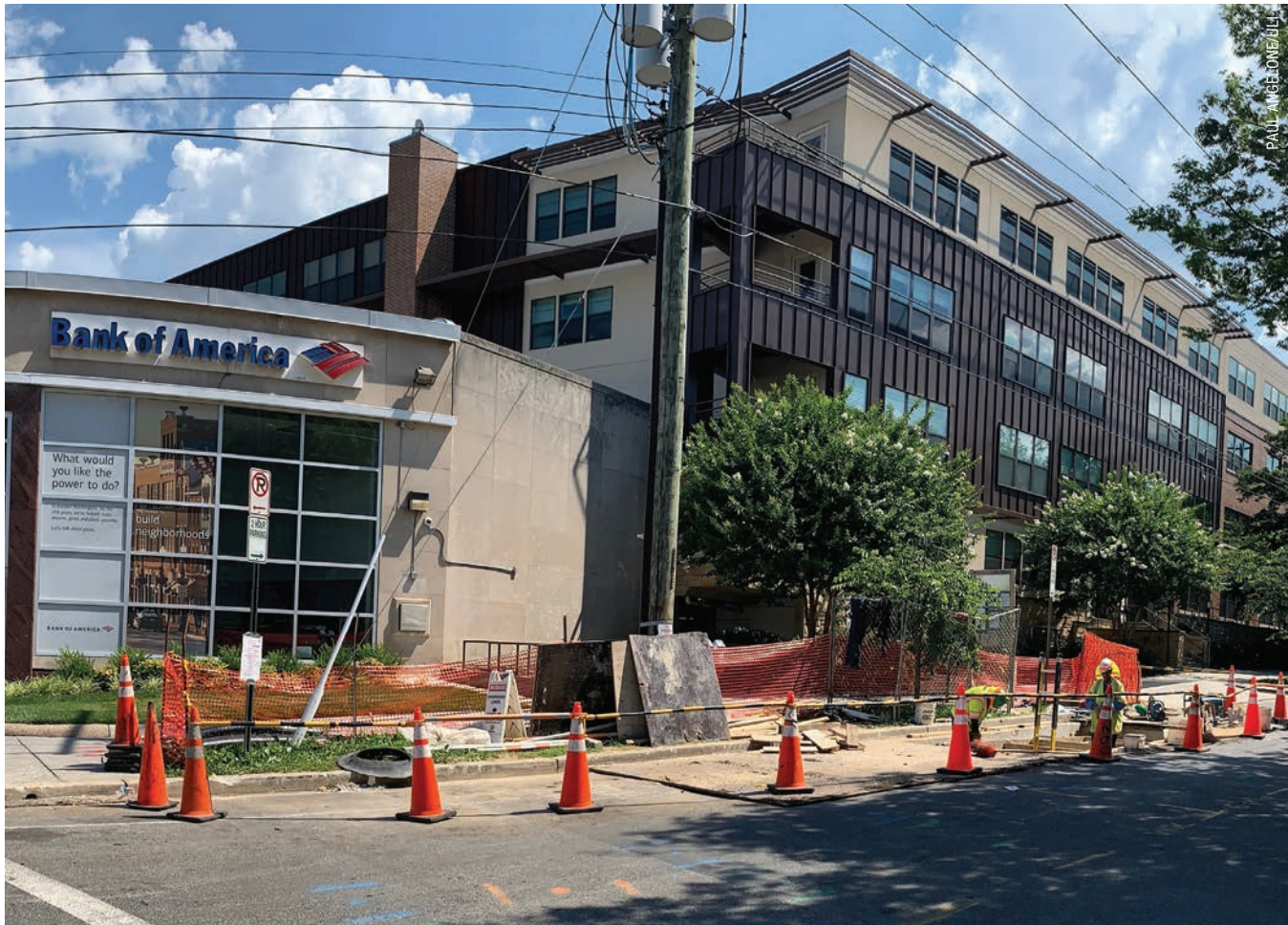
New multifamily construction near Wisconsin Avenue, N.W.
