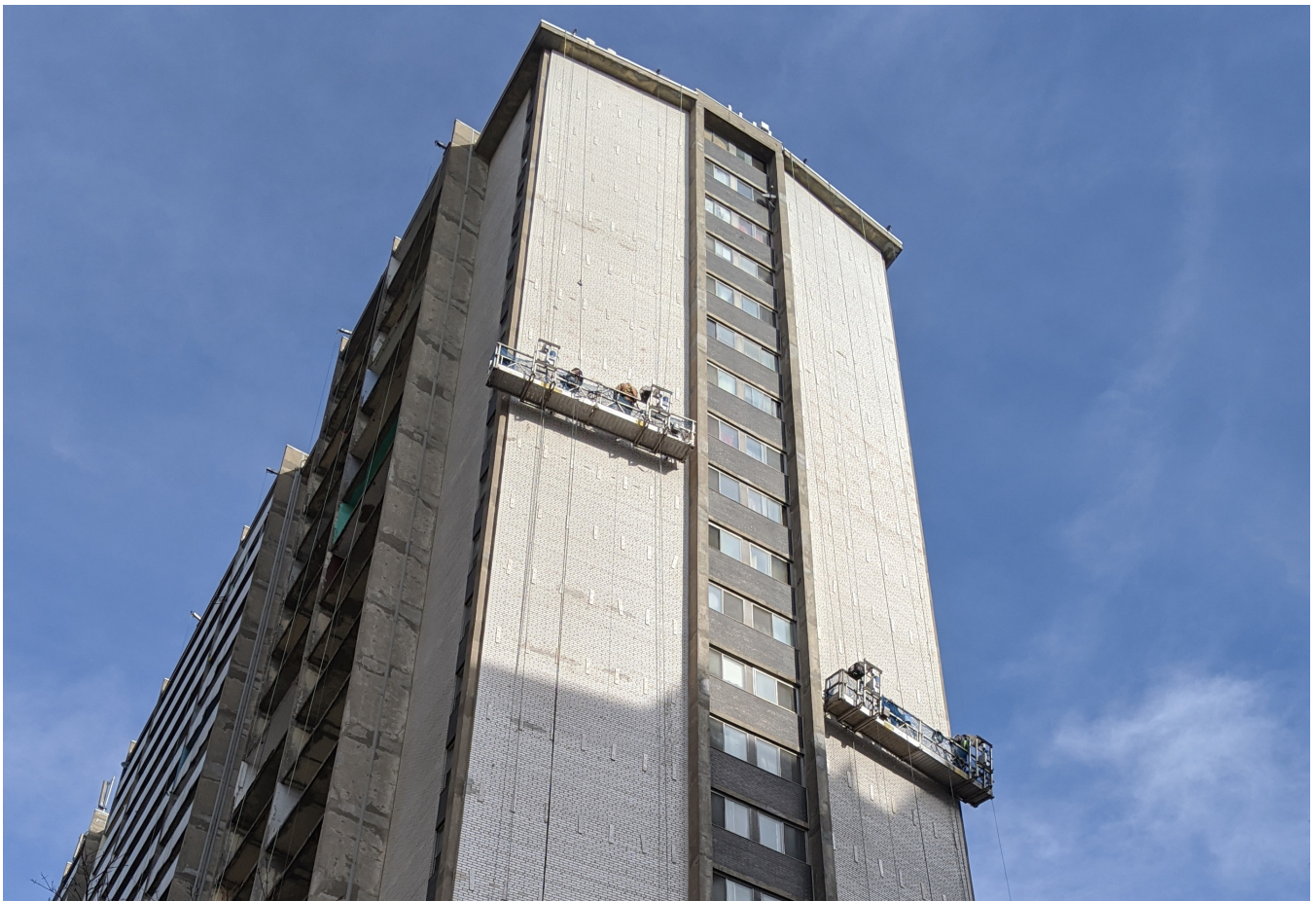
Tower refurbishment underway in St. James Town.
