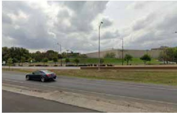
Brand visibility of the ITC building from neighboring Interstate 37 is poor.
