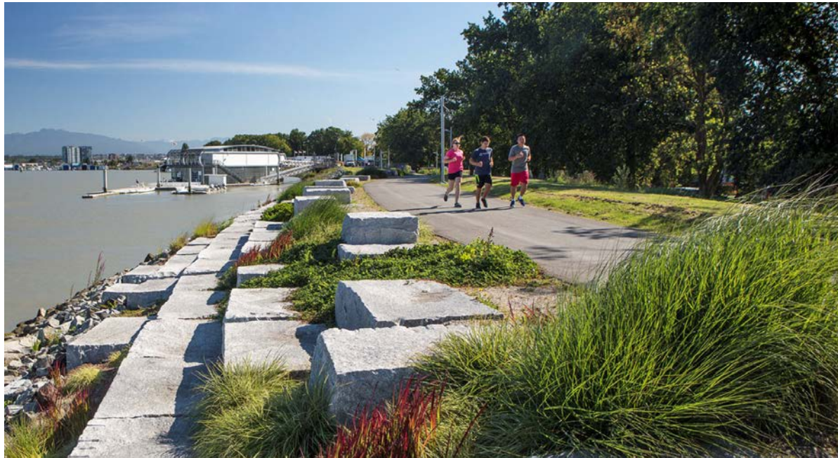
A shoreline is elevated to support a trail, but it is also stepped to provide amphitheater-style seating.
