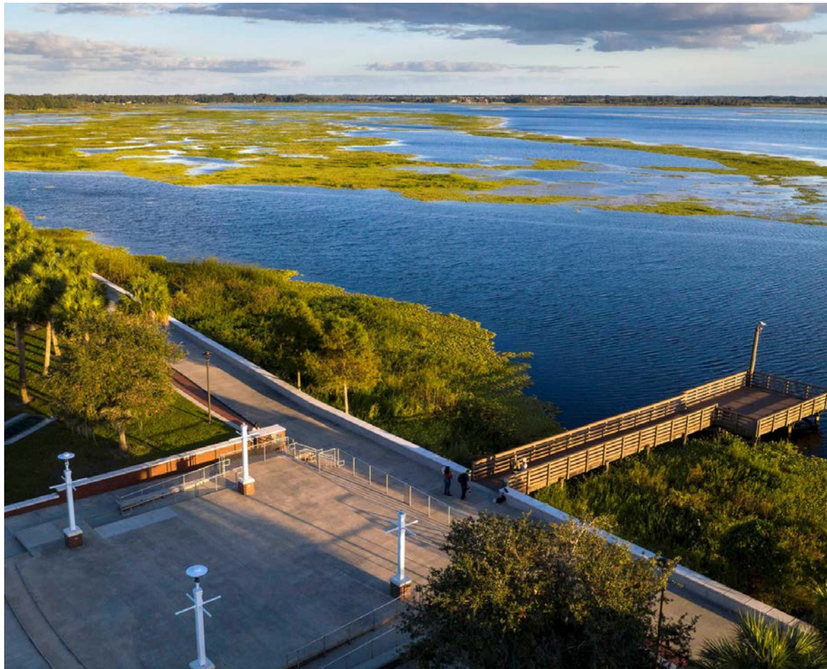
An elevated trail next to a shoreline that has been planted with vegetation that can slow and detain floodwaters.
