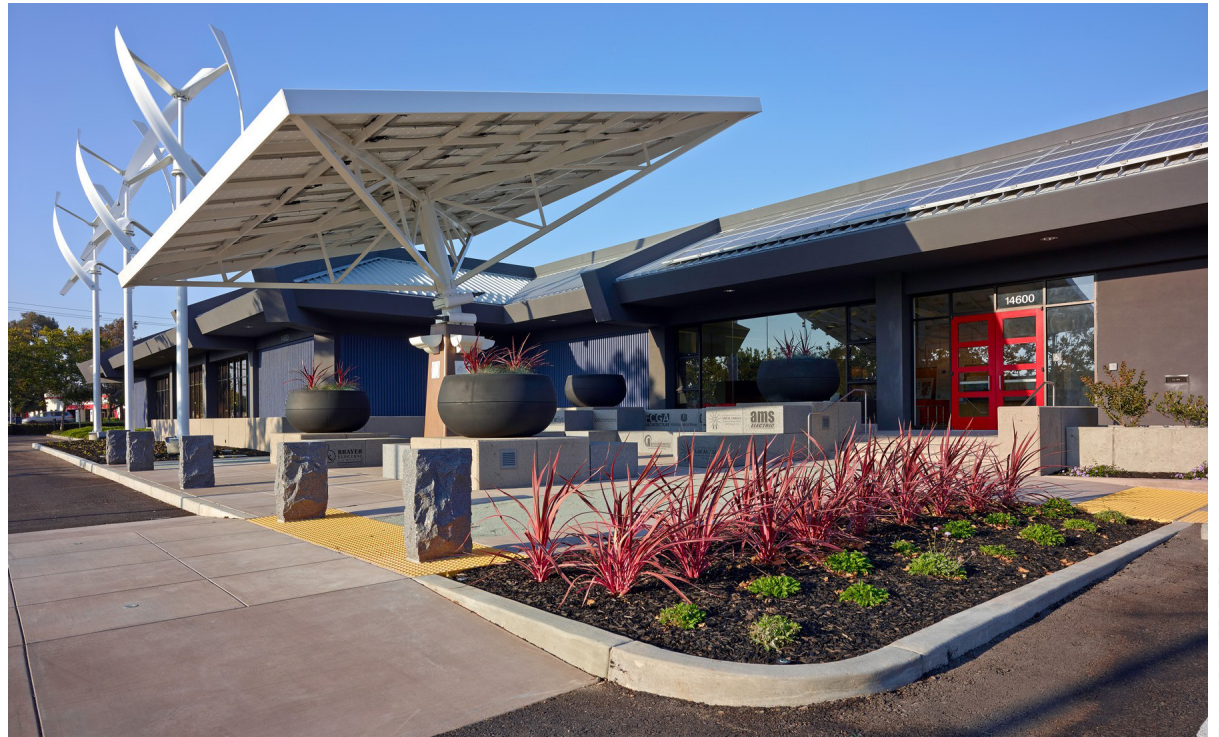
IBEW Local 595 Zero Net Energy Training Center.
