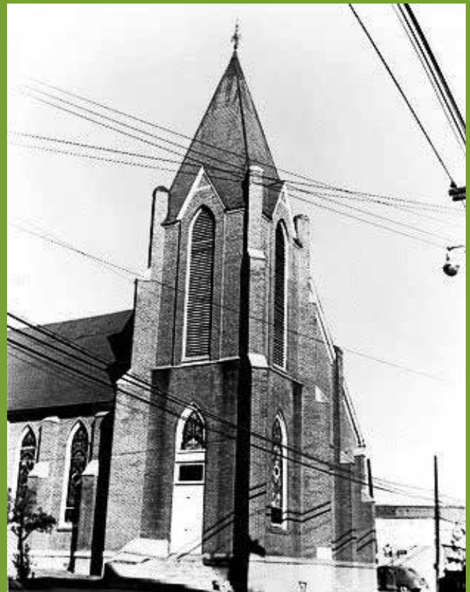
The historic St. Joseph's AME Church building, now the Hayti Heritage Center, has long been an important monument in Durham.
