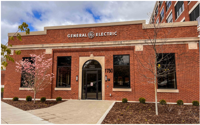
The General Electric logo is still posted on the new Electric Works building, showing the appreciation for the history of GE and its impact on the city's workforce.
