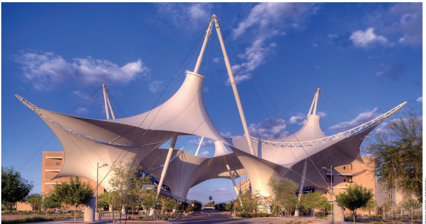
This public art installation at the heart of SkySong offers an iconic gateway to the Scottsdale Innovation Center and shade during full-sun days.
