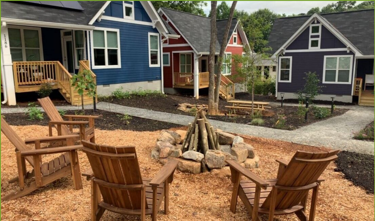
The Cottages at Vaughan consists of eight micro-cottage homes clustered around a common green space.
