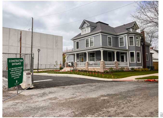
A home adjacent to construction in the Southeast neighborhood of Fort Wayne.
