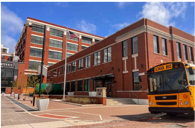
AMP Lab is a program that brings high school students from diverse backgrounds to Electric Works for half-day sessions full of real-world experience in an innovative environment.
