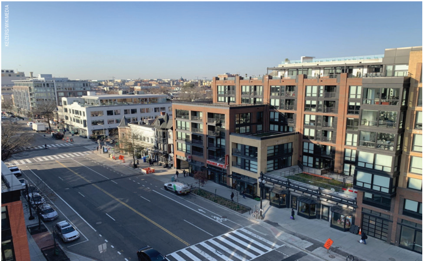
Mixed-use development on 14th Street, N.W., in Washington, D.C. A similar mixed-use approach could be used for a catalytic project within the study area.
