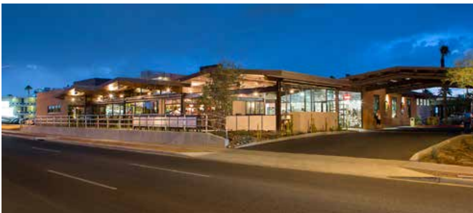
The sawtooth roof, as viewed from Camelback Road.
