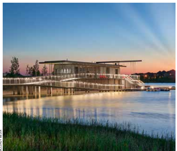
A new boathouse sits high above the shores of Josey Lake, allowing the water level to fluctuate naturally.
