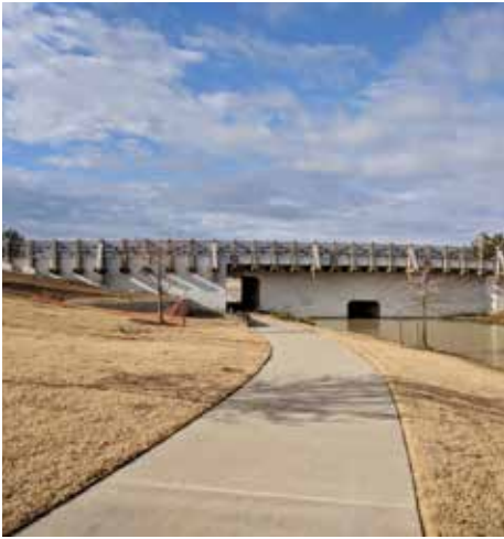
Culverts allow pedestrians and paddlers to pass, while managing the rate of stormwater flows.
