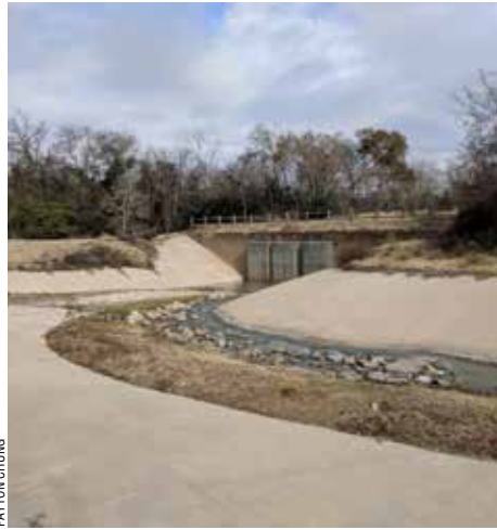
A single outfall channel connects Josey Lake and Cypress Lake through a levee to Cypress Creek. A mountain bike trail runs atop the wooded levee.
