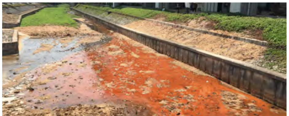
Effluent overflows into the Dasha River
