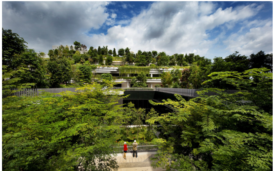
Kampung Admiralty's rooftop gardens
