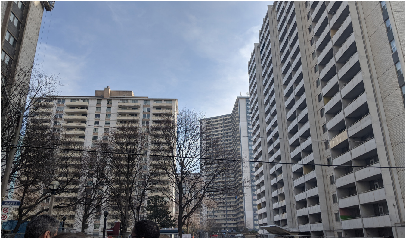
Achieving scale with retrofits is important to drive market transformation.
