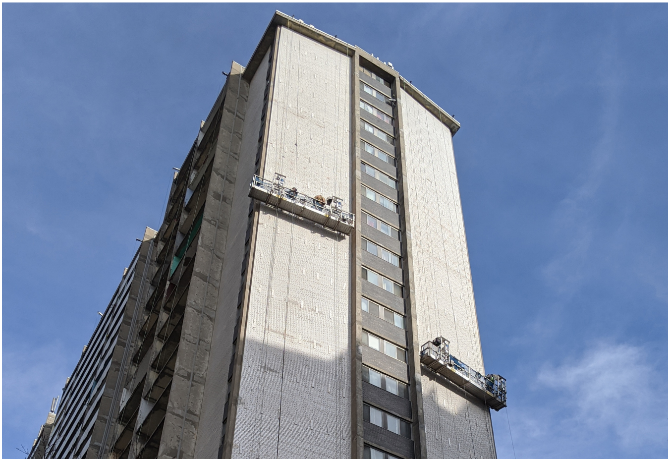
Tower refurbishment underway in St. James Town.
