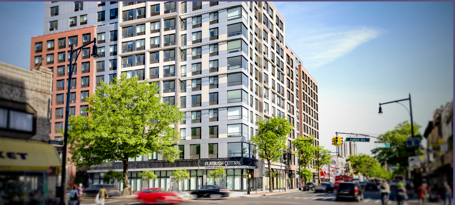
The NYC Department of City Planning consulted on the design of the 14-story building to include setbacks and different facade treatments to make the feel less imposing. (BRP Caton Flats LLC)
