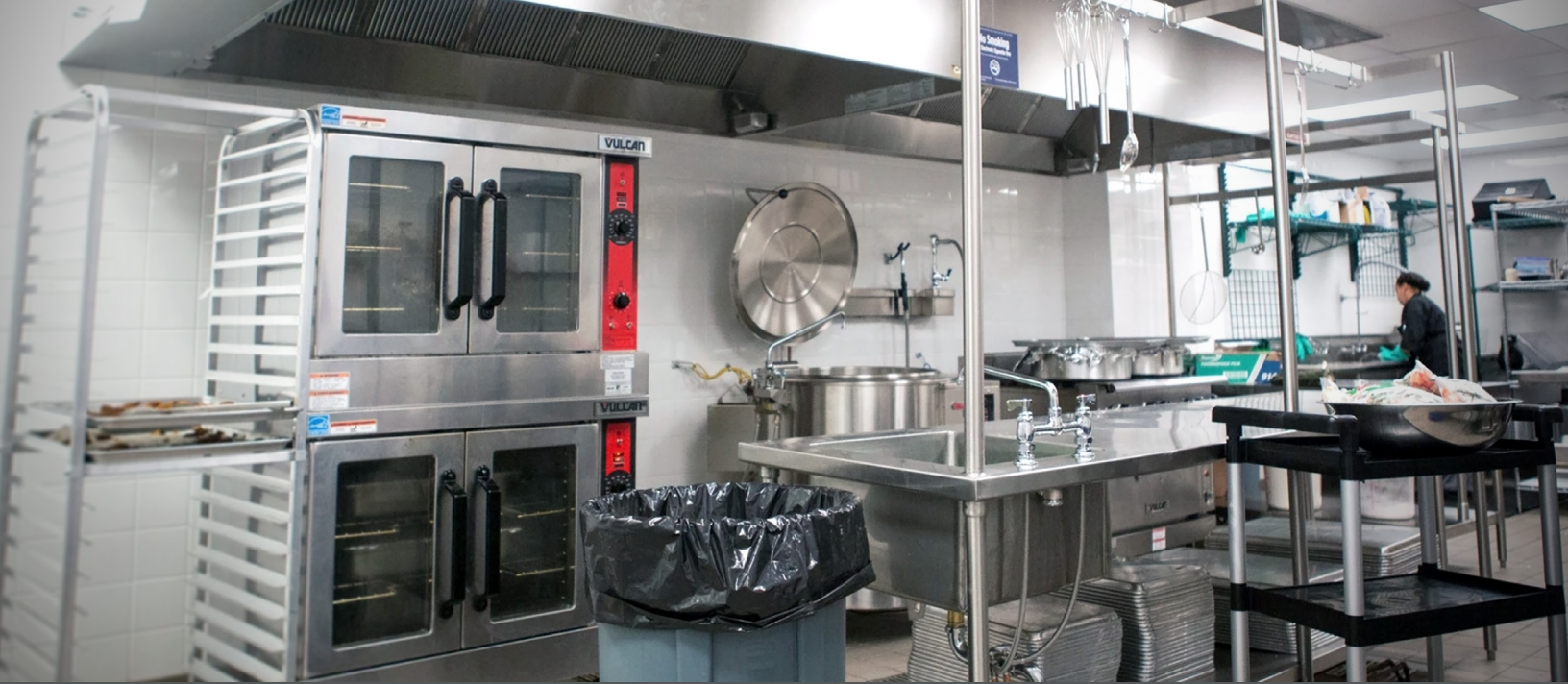
The shelter includes kitchen facilities. (Courtesy of BRC)
