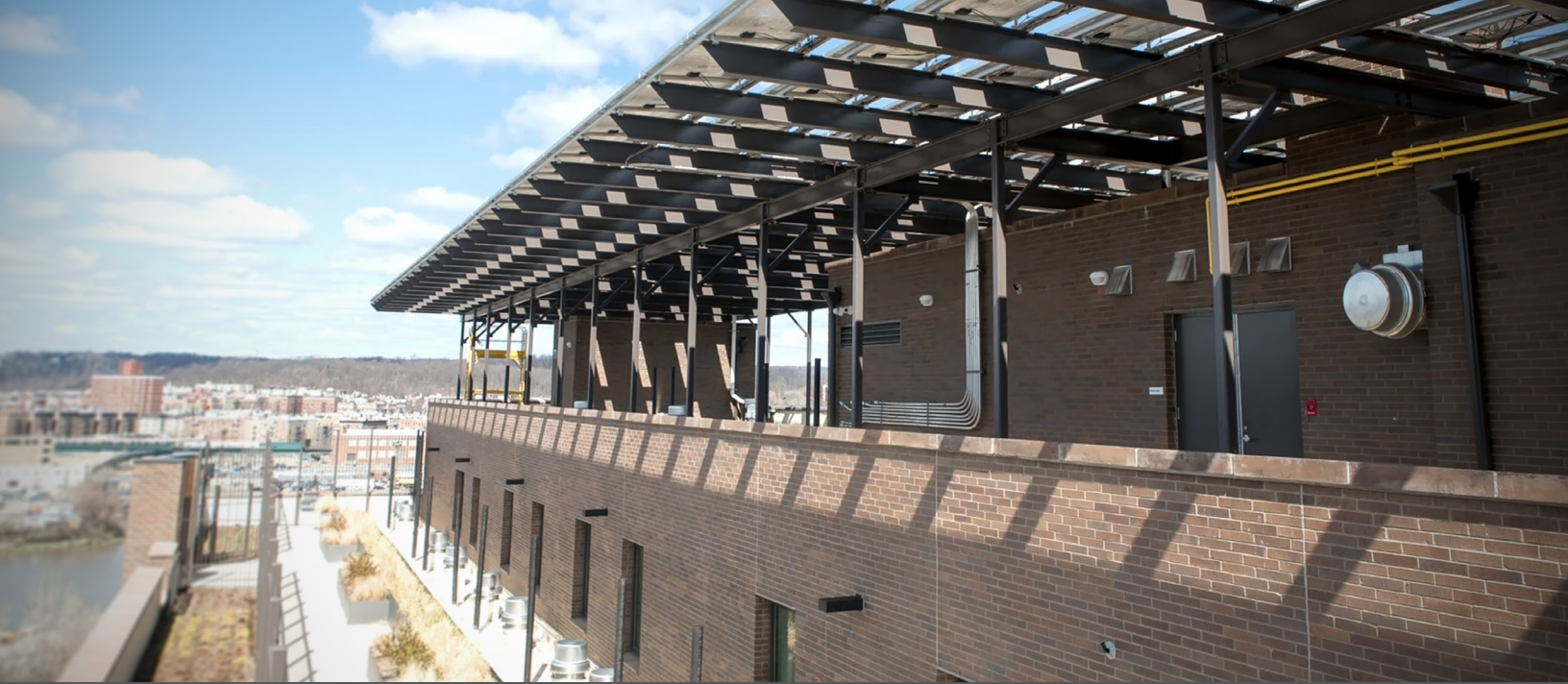
The Landing Road complex includes solar panels for energy efficiency. (Courtesy of BRC)
