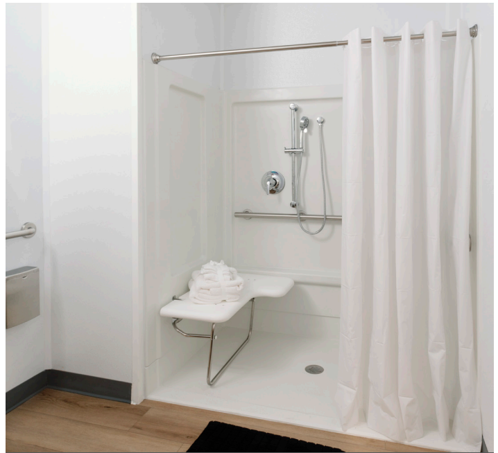
ADA-accessible roll-in showers include a folding shower seat, a grab bar, and shower controls with a handheld shower head. (Courtesy of Gregg Willett)
