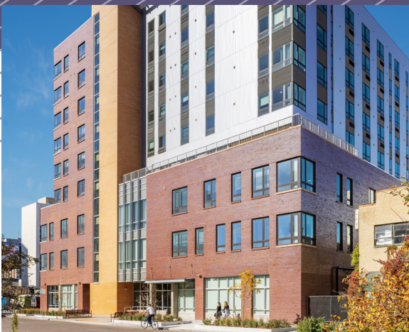
Facade of the John Parvensky Stout Street Recuperative Care Center and Renaissance Legacy Lofts. (Courtesy of Frank Ooms)
