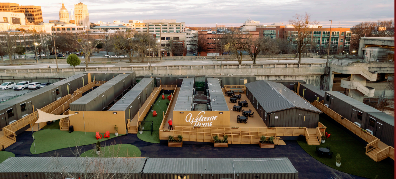
The Melody project site displays the layout with the housing facilities (former shipping containers), outdoor spaces with seating and decor, green spaces, and the surrounding neighborhood. (Courtesy of The Beck Group)
