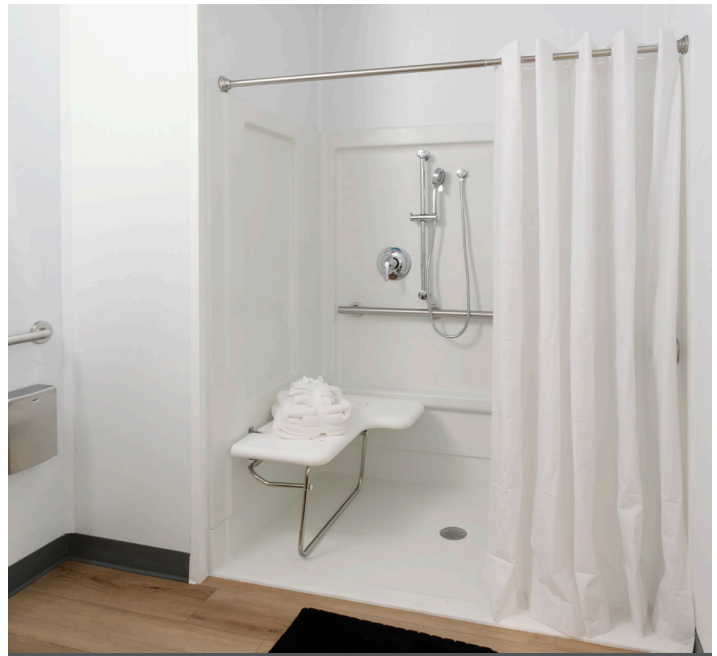
ADA-accessible roll-in showers include a foldable shower seat, a grab bar for support, and shower controls with a handheld showerhead. (Courtesy of The Beck Group)
