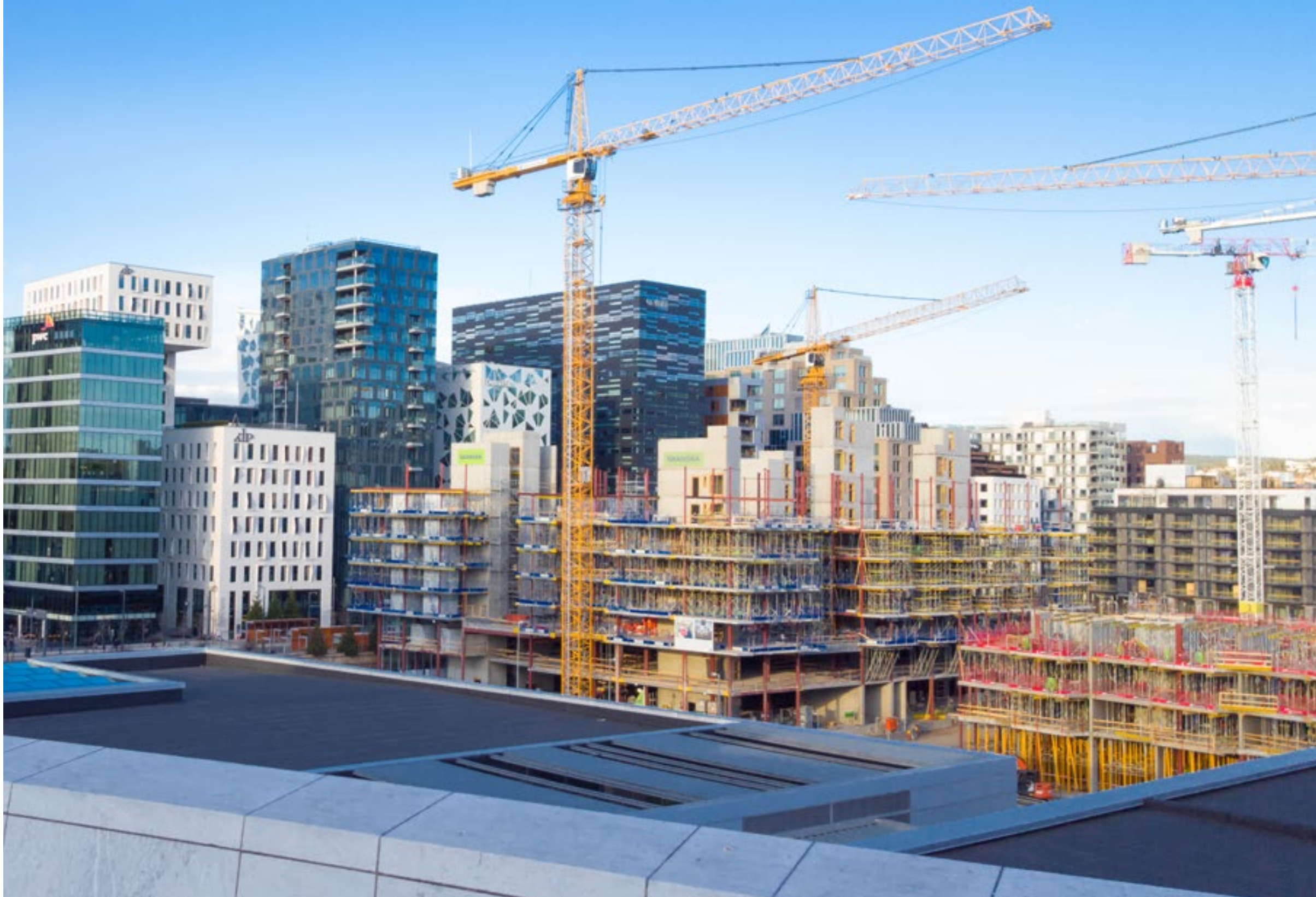
CONSTRUCTION IN OSLO, NORWAY
