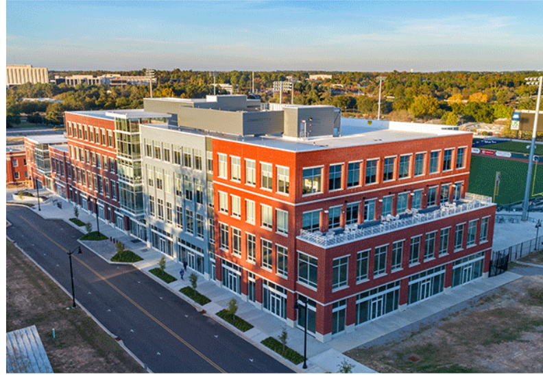
First Base Building in the BullStreet District of Columbia, South Carolina.
