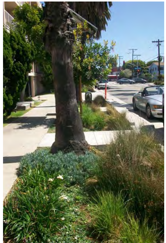
The city of Santa Monica modified a section of Bicknell Avenue with bioswales and permeable pavement to collect urban runoff before it entered the storm drain system.
