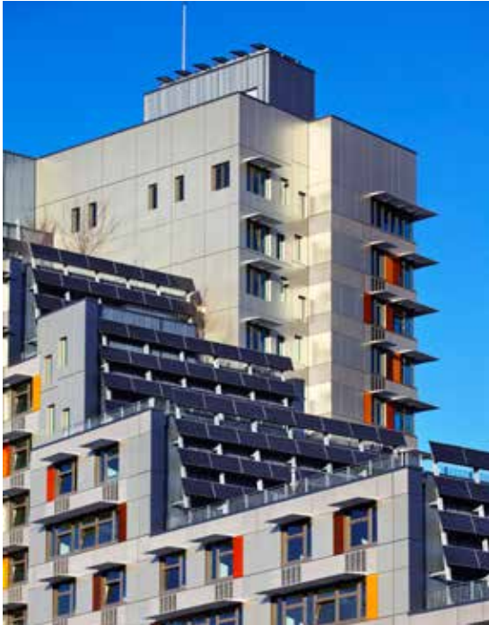
Solar panels on the Via Verde, the Bronx, New York.
