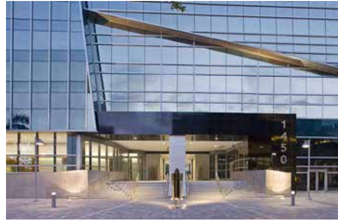
The Brickell Avenue entrance lobby is raised several feet above the street level and the floodplain.
