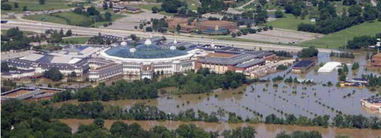
An aerial view of flooding at the Grand Ole Opry House. The Tennessean
