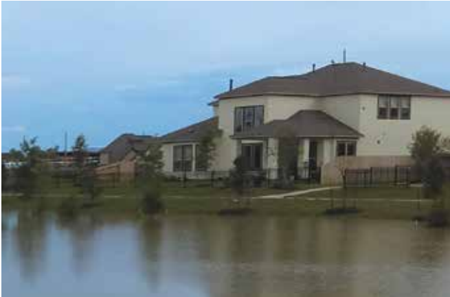
Stonebrook Estates' natural drainage system managed the waters from the Tax Day Flood of 2016, which severely affected Houston. (Terra Visions LLC)
