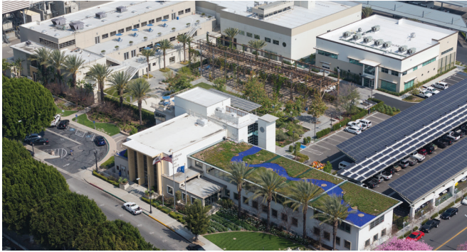
An aerial view of Burbank Water and Power shows the dynamic campus, which includes green roofs, solar panels, and an interior courtyard. (Sibylle Allgaier, Heliphot)
