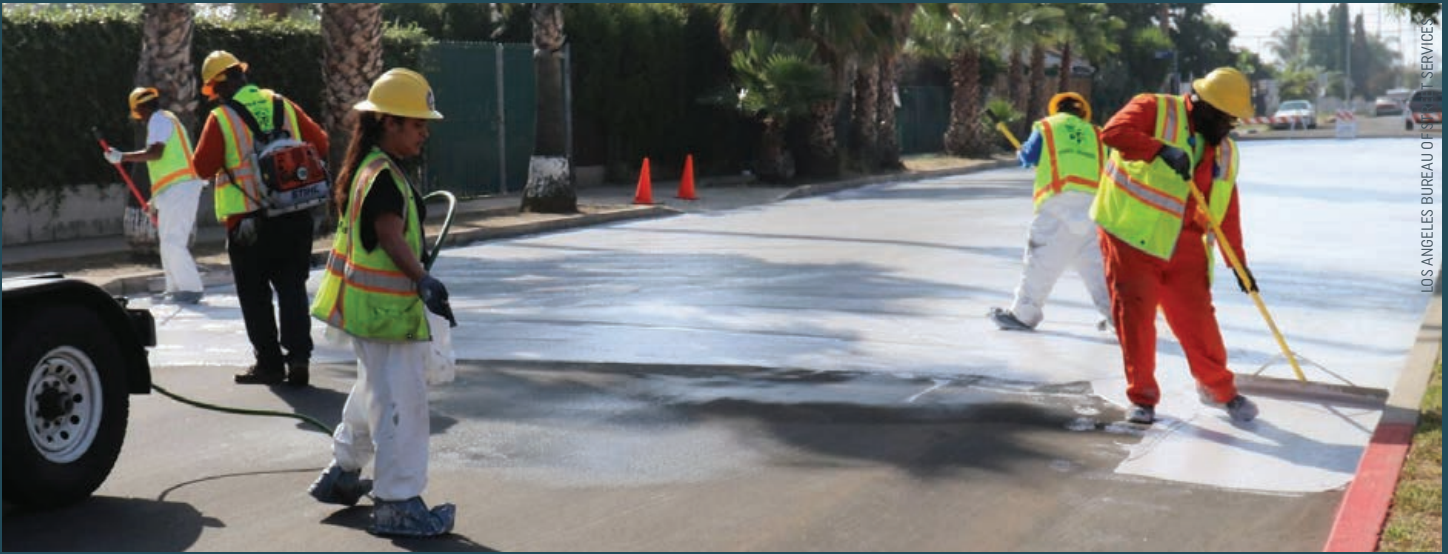
Pilot tests in Los Angeles demonstrate both benefits and challenges of cool pavement. The city is continuing to evaluate, refine, and expand this heat-mitigation technique.
