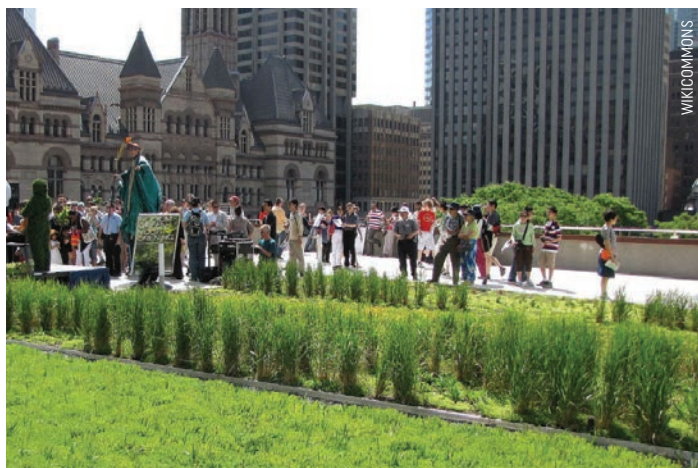
After passing the Green Roof Bylaw, Toronto installed the city's largest publicly accessible green roof atop City Hall.
