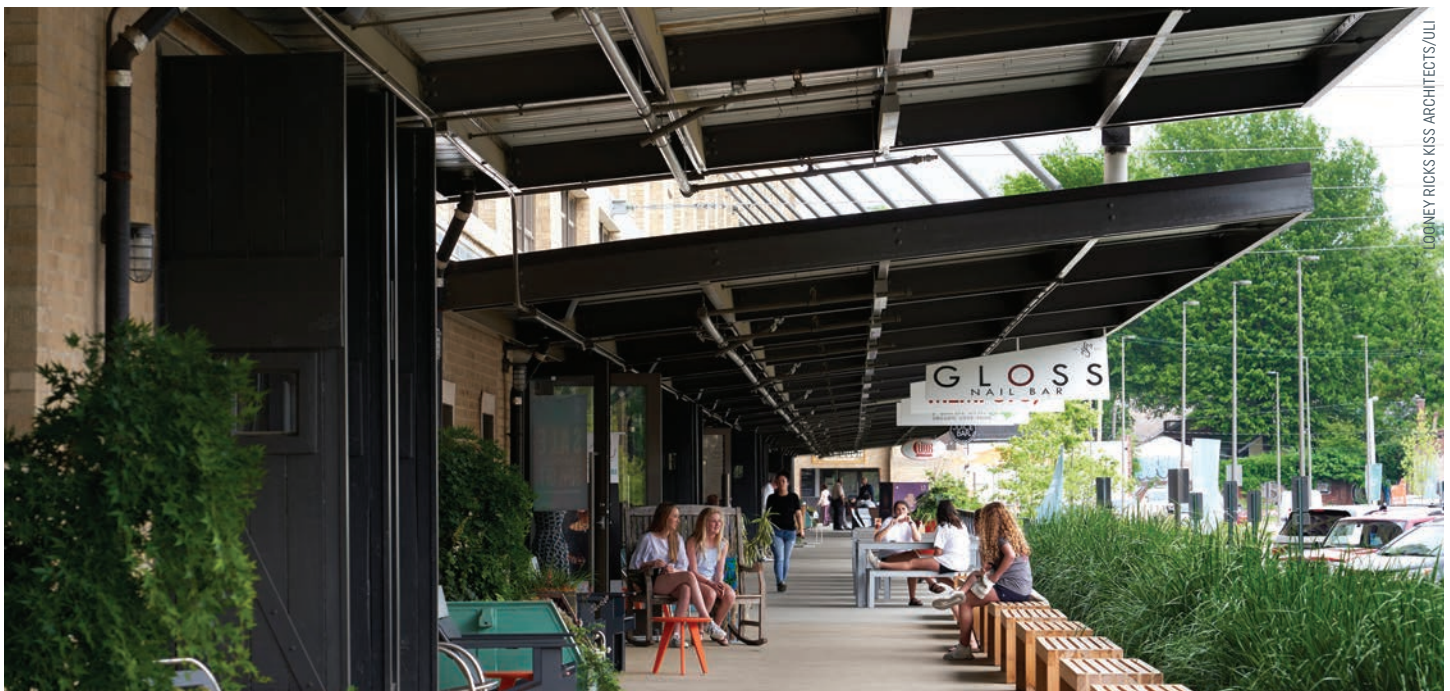
Deliberate efforts to prioritize efficient mechanical equipment to reduce long-term operating costs at Crosstown Concourse (Memphis, Tennessee), one of the world's largest historical adaptive use LEED Platinum buildings, paid off, achieving an energy cost savings of $1.3 million.
