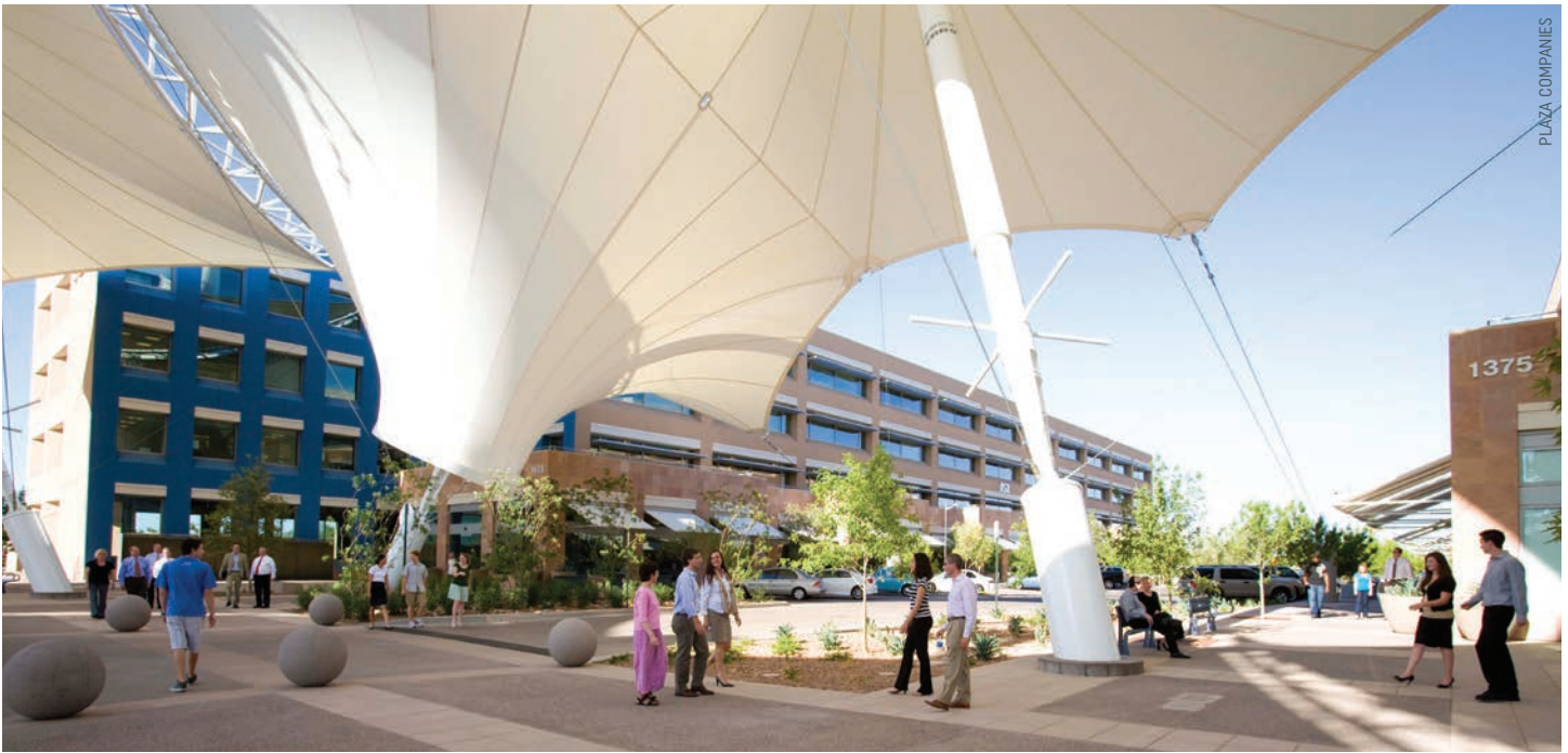
An iconic 125-foot-tall shade sail at SkySong, the Arizona State University Innovation Center, anchors the 42-acre development and is part of a heat-conscious design that helps attract tenants and reflects the founding partners' forward-thinking, entrepreneurial vision.
