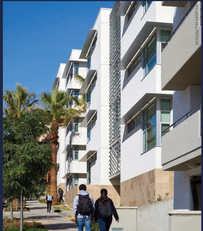
Custom housing prototypes with central courtyards, open breezeways, and operable windows help maximize shade, ventilation, and energy efficiency at Edison Eastlake.
