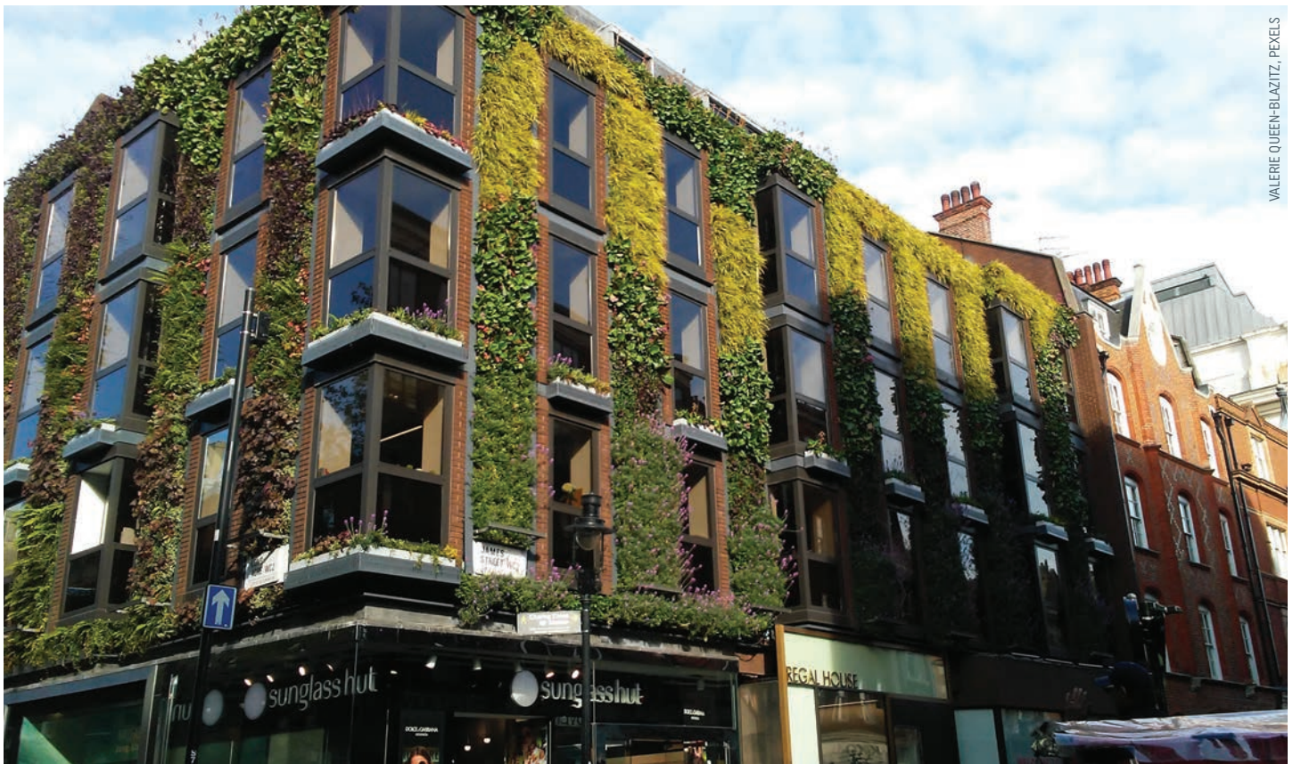
Through policies and incentives, cities can create opportunities for developers to implement heat-conscious design elements like green walls.
