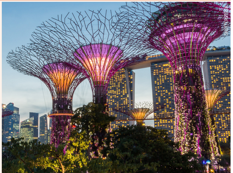
Inventive 'supertrees' attract visitors and are a cooling strategy, shading underlying recreation spaces and venting waste heat from a nearby building away from pedestrians.
