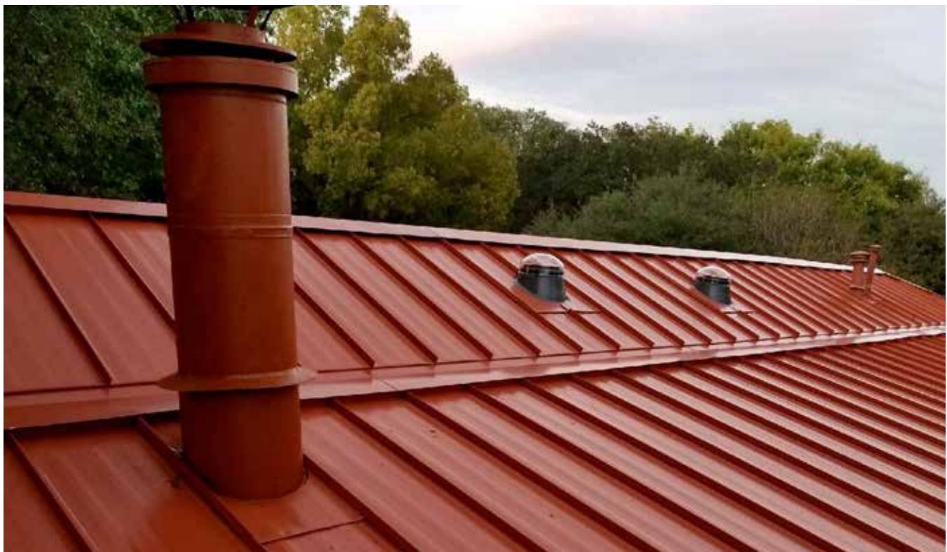
Features like steep roofs to dislodge embers and ignition-resistant materials can be required by building codes to help structures survive wildfires at higher rates. California's Building Code Chapter 7A, implemented in 2008, is widely regarded as a best-in-class wildfire resilience measure.
