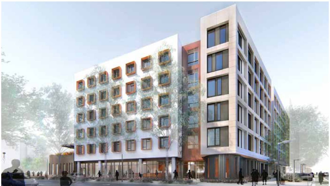
Maceo May, a 105-unit, all-electric residential development in San Francisco, is designed with an energy recovery ventilator with a MERV 13 filter, operable windows, and ceiling fans for every residential unit as well as a community space powered by on-site solar to maintain indoor air quality and continue operations during wildfires, heat waves, and power outages. Read more at developingresilience.uli.org/ .
