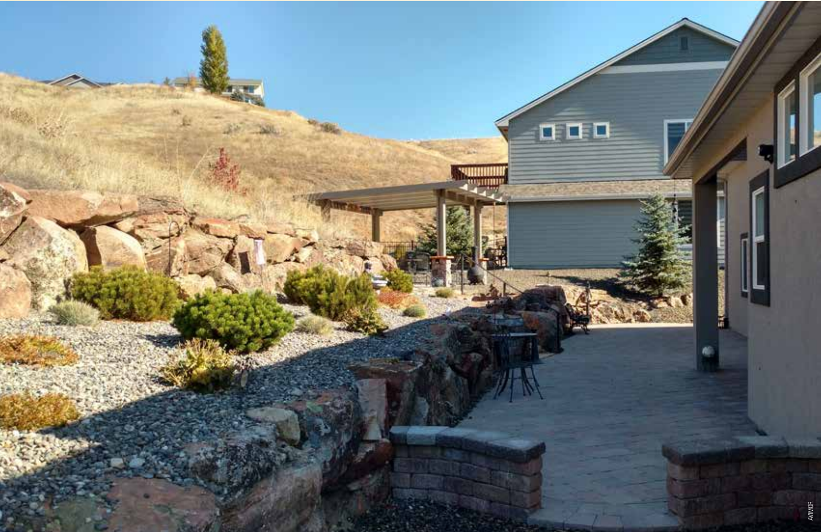
Houses at Avimor have ignition-resistant cementitious siding, class A roofs, and Firewise-approved landscaping.
