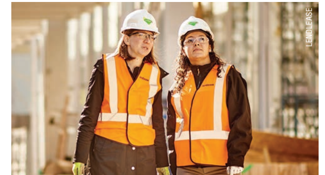
Lendlease construction site.
