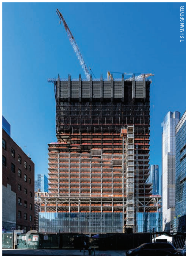
Construction underway on The Spiral.
