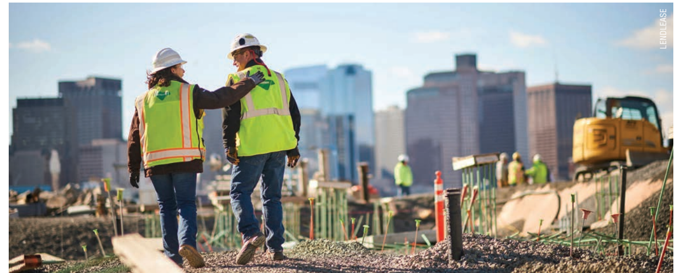
Lendlease construction site.
