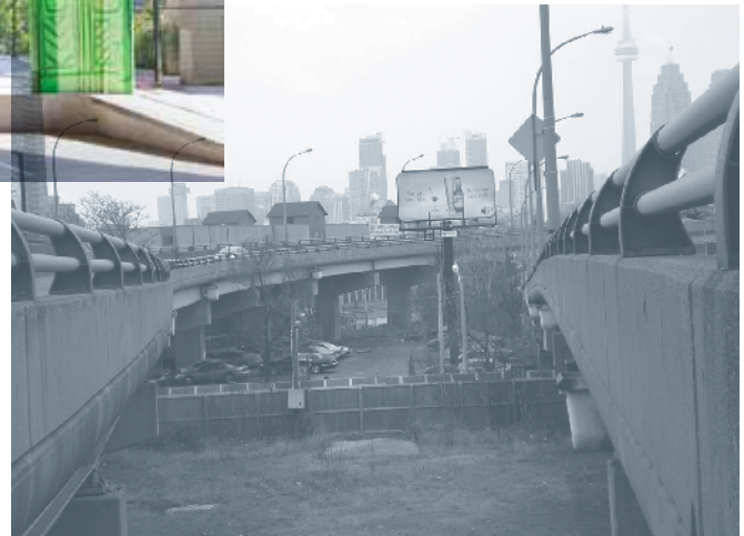
Pillars from the overpasses are an important part of the design of Underpass Park, which blends murals, lighting, and small green pockets in the formerly neglected space underneath several elevated roadways.
