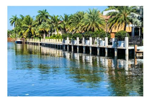
meets the four feet NAVD88 minimum and can structurally support up to 5.7 feet NAVD88 in the future.
