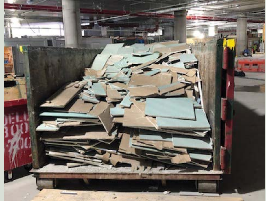
On-site source separation of drywall scrap material. (Lendlease)
