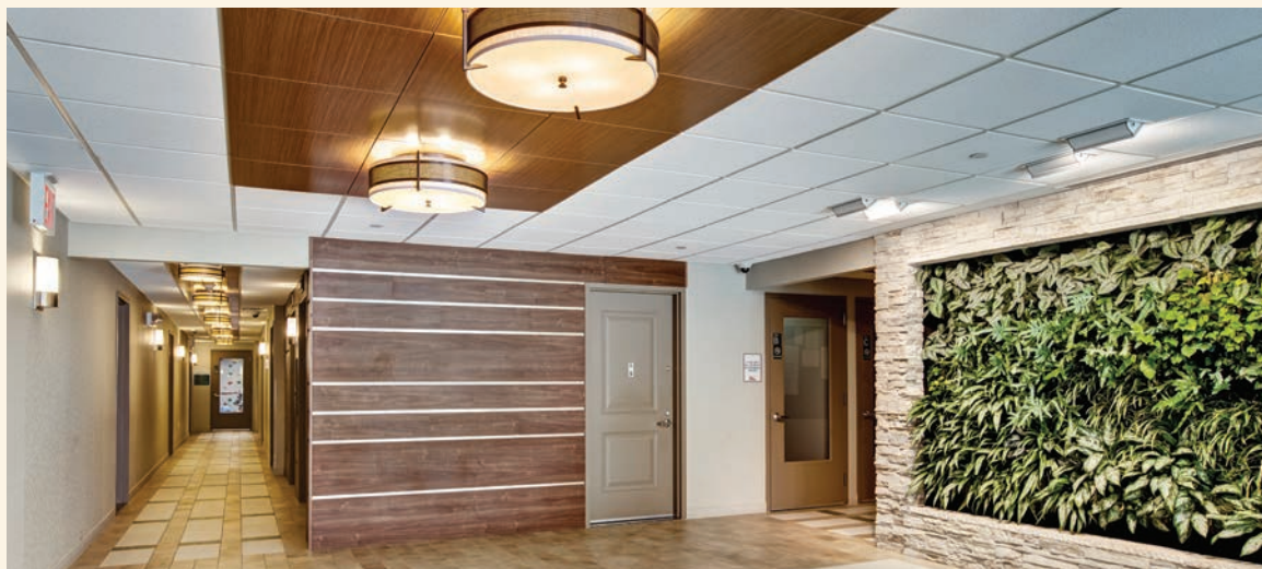
The living green wall at Arbor House—a low-income multifamily housing development in the South Bronx, New York—was designed as part of the building's LEED Platinum certification to help maintain healthy indoor air quality and reduce residents' asthma rates.
