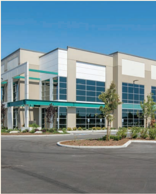
Prologis Park Tacoma was the first WELL-certified logistics facility in the world.
