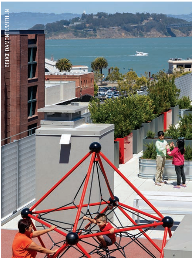
Sansome and Broadway Family Housing provides affordable housing for families, including formerly homeless families, in the heart of San Francisco.
