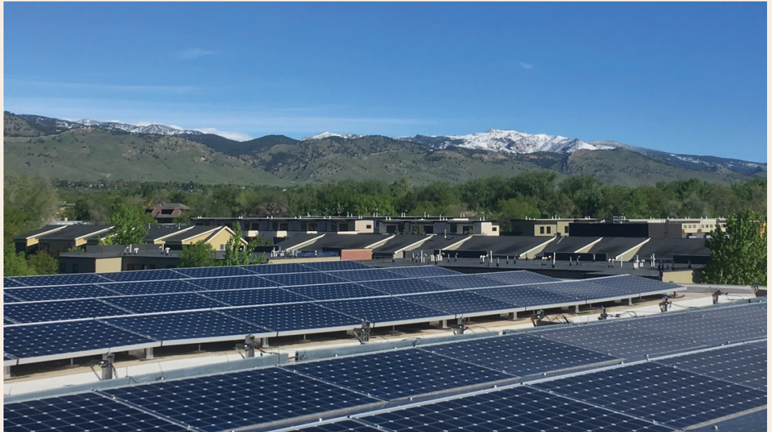
Boulder Commons roof with solar panels. (Morgan Creek Ventures)
