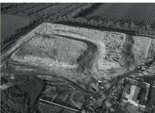
Hazardous waste landfills can pose risks to nearby communities.
