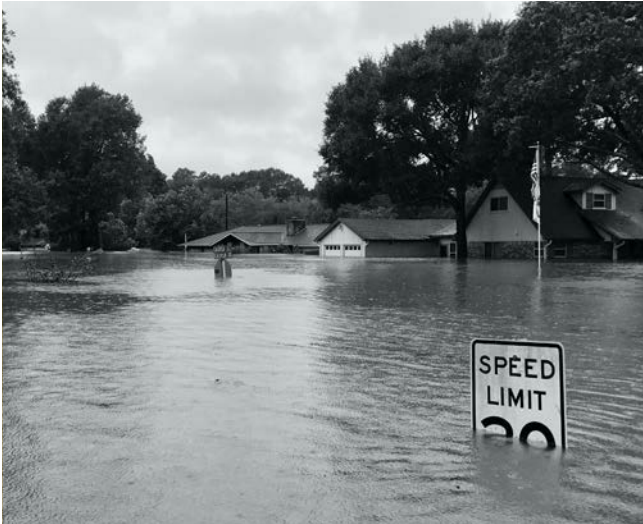
Flooding in Houston caused by Hurricane Harvey.
