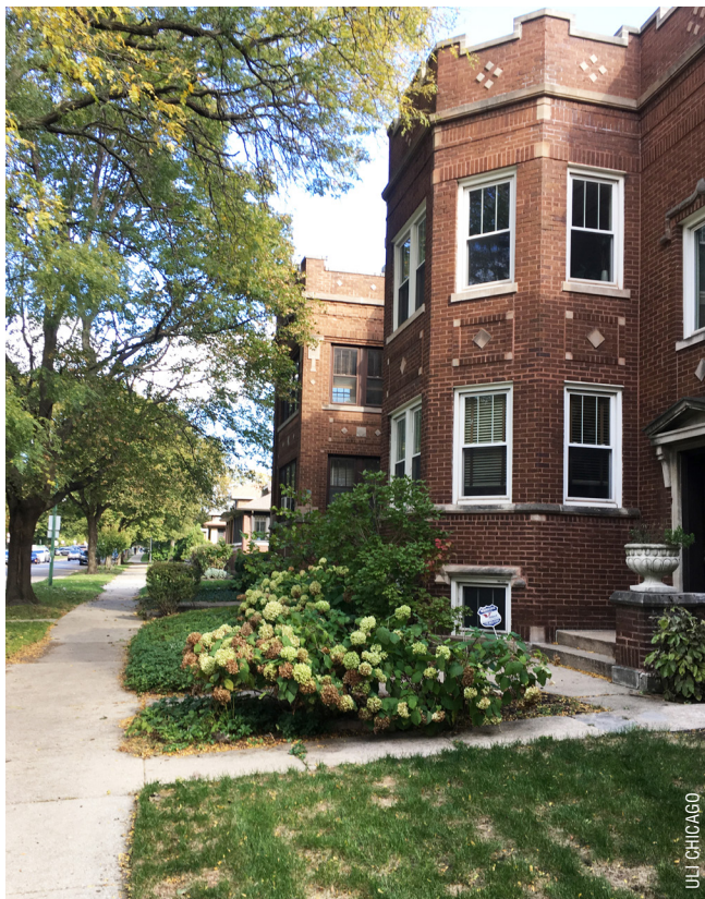
Older two-flats and four-flats make up a significant portion of Chicago's residential building stock.
