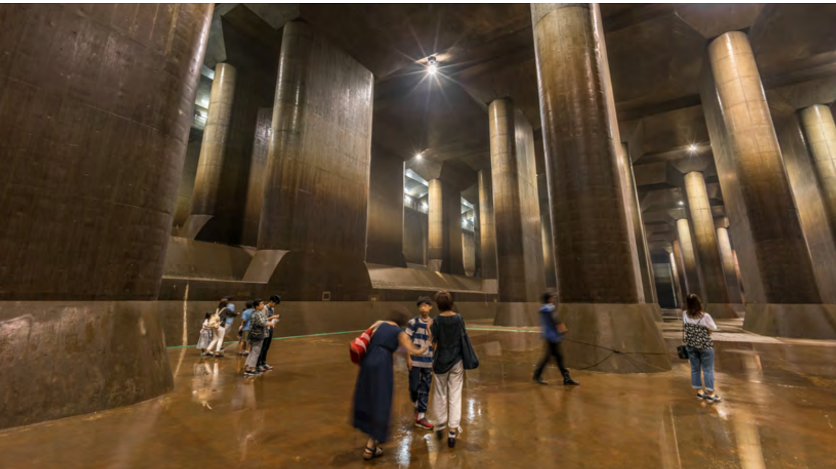
The Greater Tokyo Outer Area Discharge Channel is the world's largest underground flood control facility. (Manuel Ascanio/Shutterstock)
