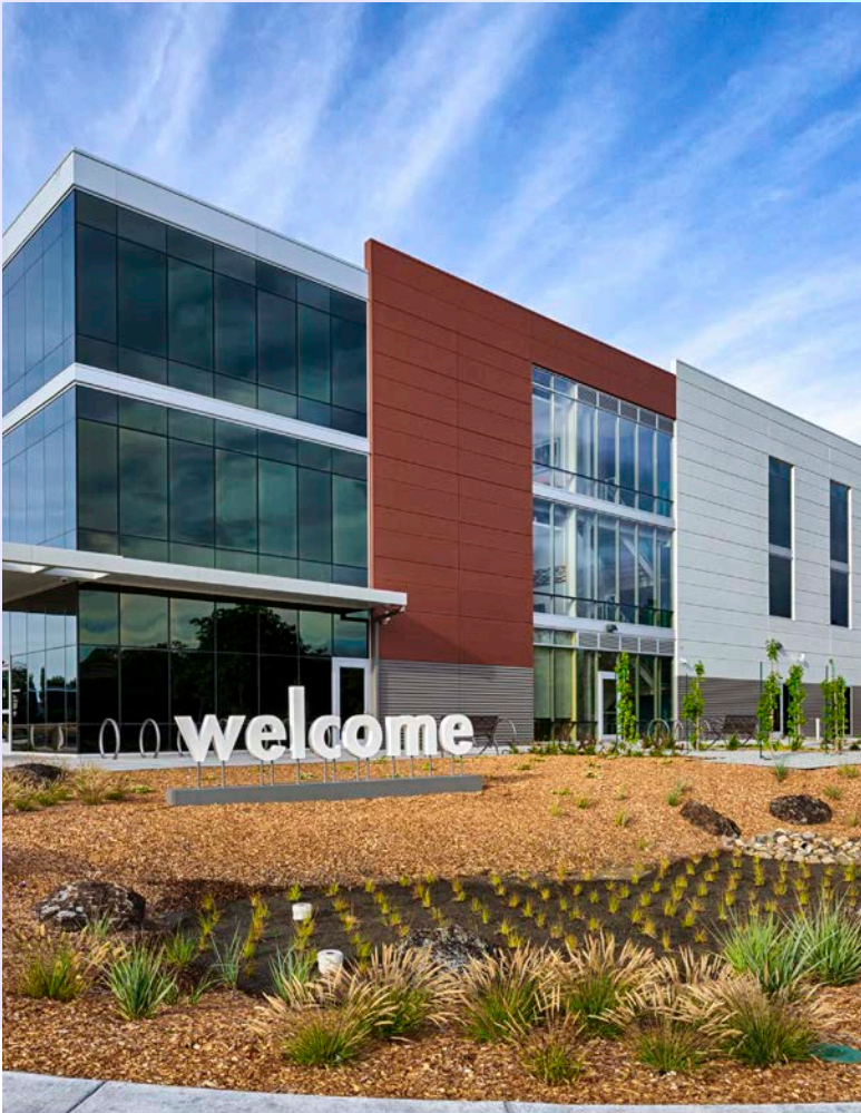
Kaiser Permanente's all-electric Medical Office Building in Santa Rosa, California.
