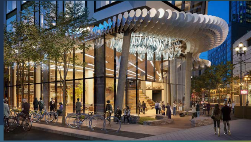
Entrance to offices at 30 Van Ness.
