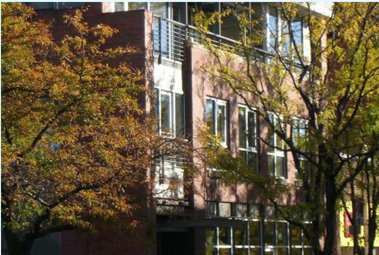
A 2003 LEED Platinum all-electric retrofit in Boulder, Colorado, by Morgan Creek Ventures.
