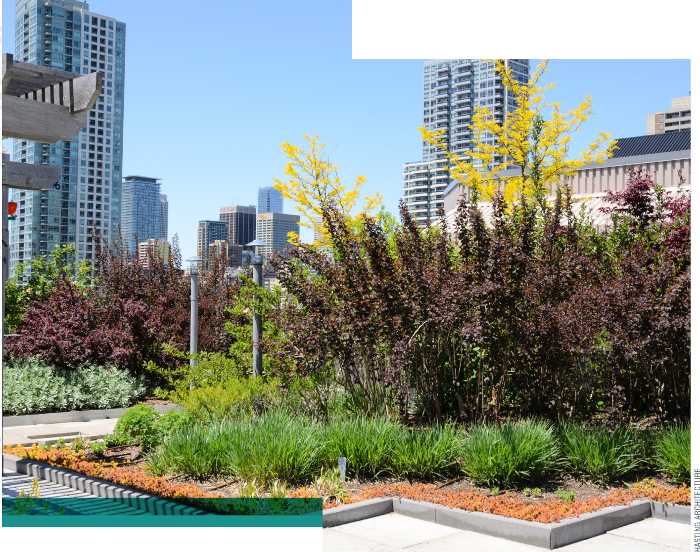
This building rooftop features a variety of green roofing materials, cooling the building while also capturing and using rainfall that would otherwise be diverted into stormwater management systems.
