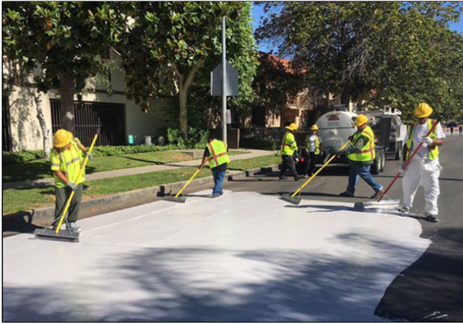
Light-colored coatings can be applied to paved spaces and streets to increase the reflectivity of the space and reduce heat absorption.
