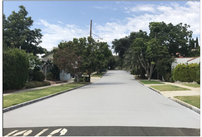
Light-colored coatings can be applied to paved spaces and streets to increase the reflectivity of the space and reduce heat absorption.
