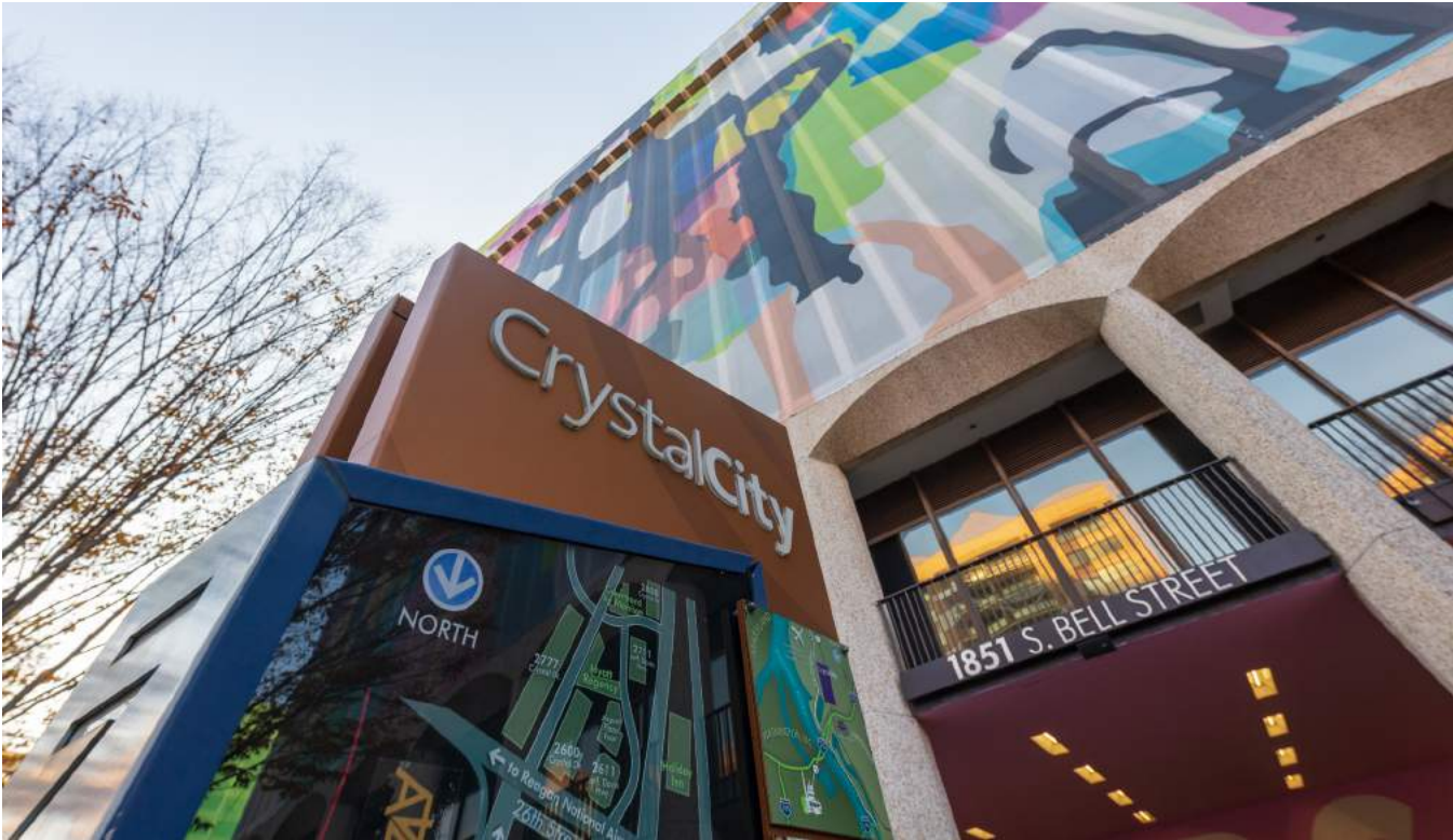
The future site of Amazon HQ2 in National Landing.
