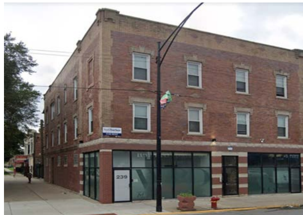
Chronically vacant ground level commercial space can be repurposed to create accessible residential units.
