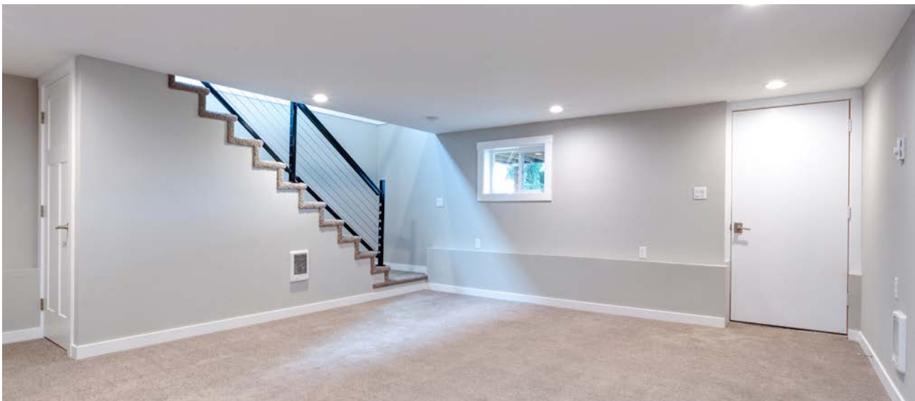
Required minimum ceiling height for basement units has been reduced to 7'-0" in the new building code (compared to 7'-6").
